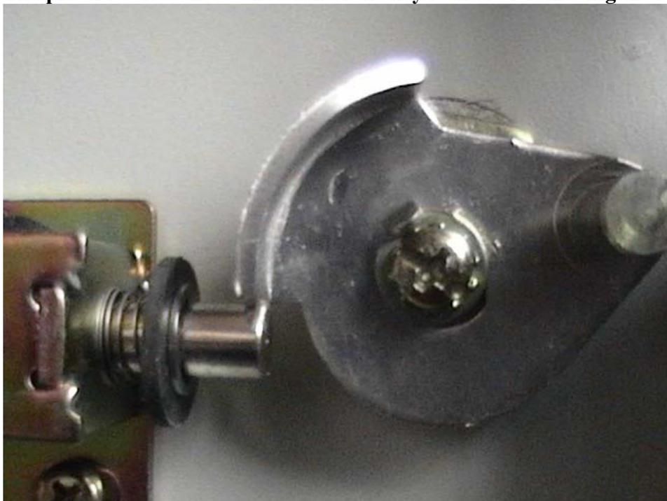
**Step two- Remove the screw holding the tailpiece on the back of the lock, to do this you need to bend the**
